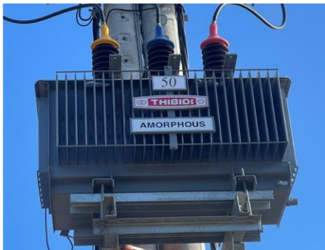
Figure 1. The model of APCTs of 50 kVA.
