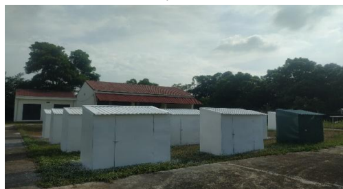
Figure 1. House samples with corrugated iron roofs coated with solar heat reflective paint.
